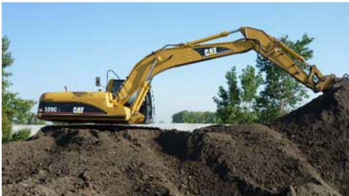
Caterpillar 320C excavator with operator $95 per hour Float charge $150.00 per hour.
